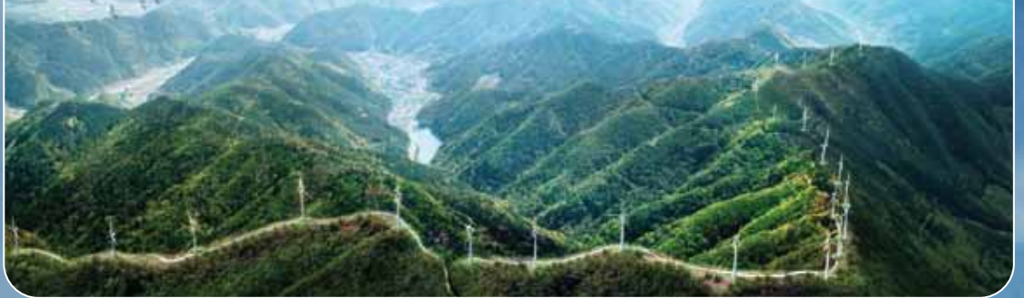
Uiryeong wind farm 18.75MW(750kW x 25Sets)
