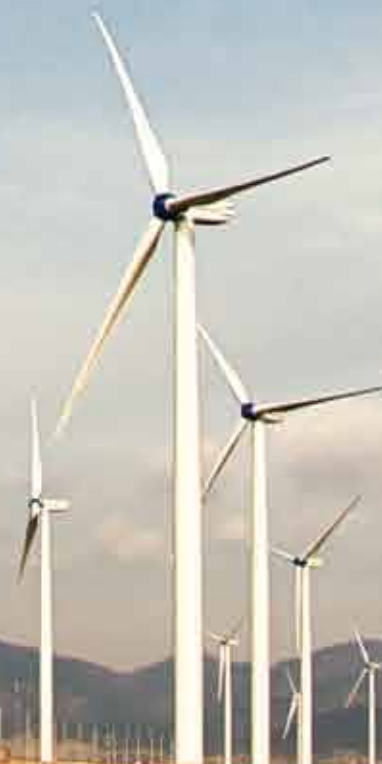
Yeongkwang Baeksu wind farm 40MW(2MW x 20Sets)
